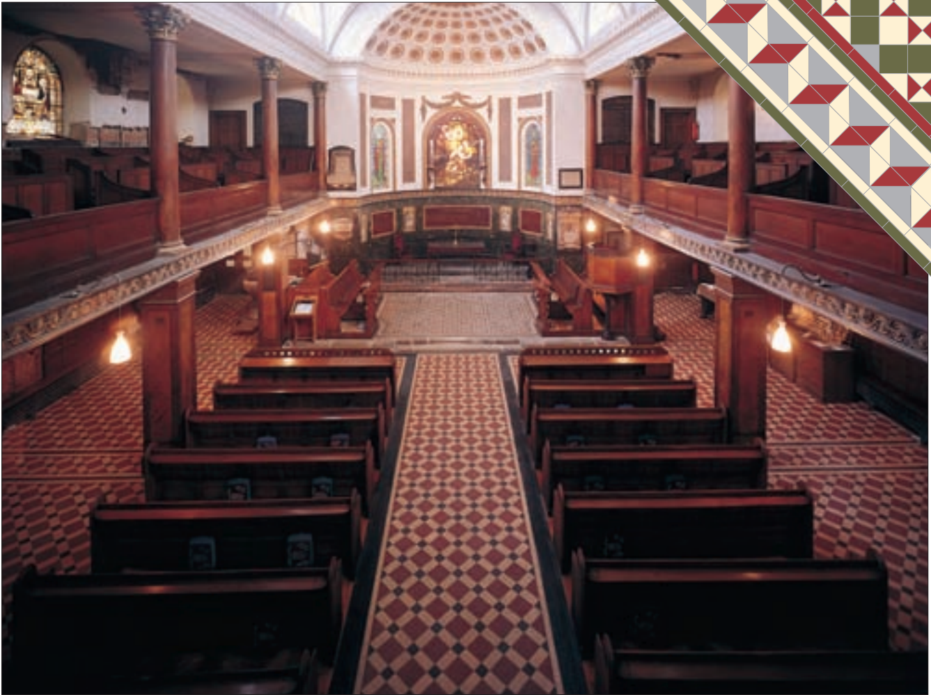
Extensive renovation work at this church included the use of Original Style tiles to replicate exactly a much damaged Victorian floor
